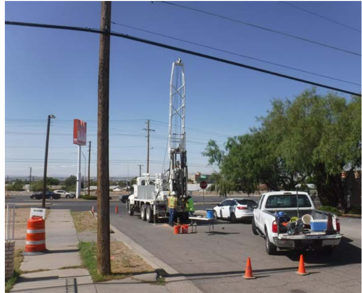
PHOTO NO. 2: General view of drilling activities at exploration vertical boring B-1 location.
